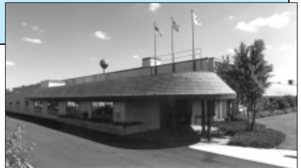
Hydraulics Division Headquarters, Eden Prairie, Minnesota
